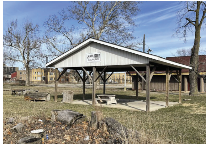
FIGURE 37: Picnic Shelter at Reed Park
